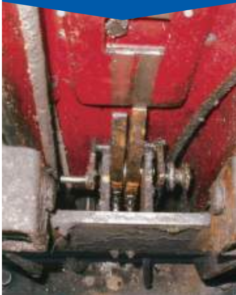
Rusty wire rope
